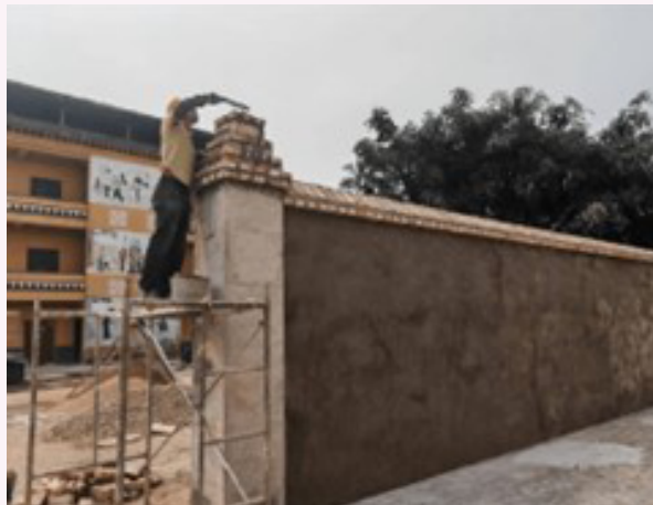
Gekui Kindergarten Renovation
