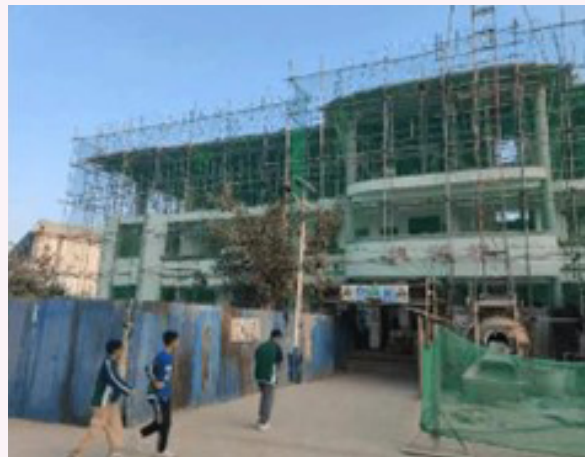
Gekui Middle School Dormitory Building Construction
